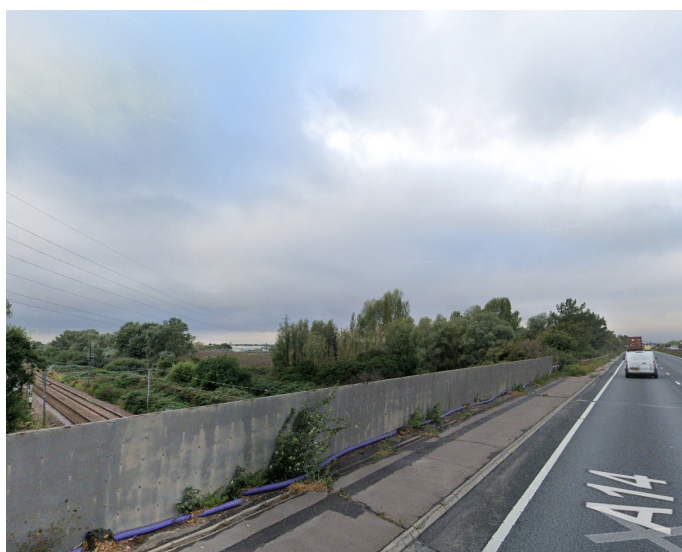
Fig. 76 A14 Highway looking onto application site
