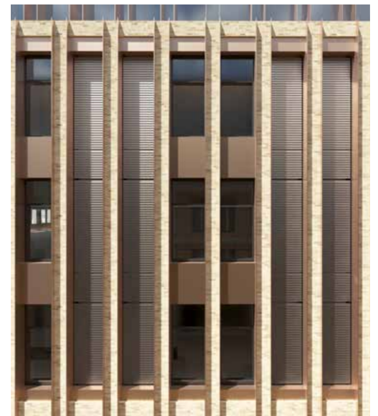
Studies showing how vertical louvres can be used as 'shadow' lines to break up the building mass.
