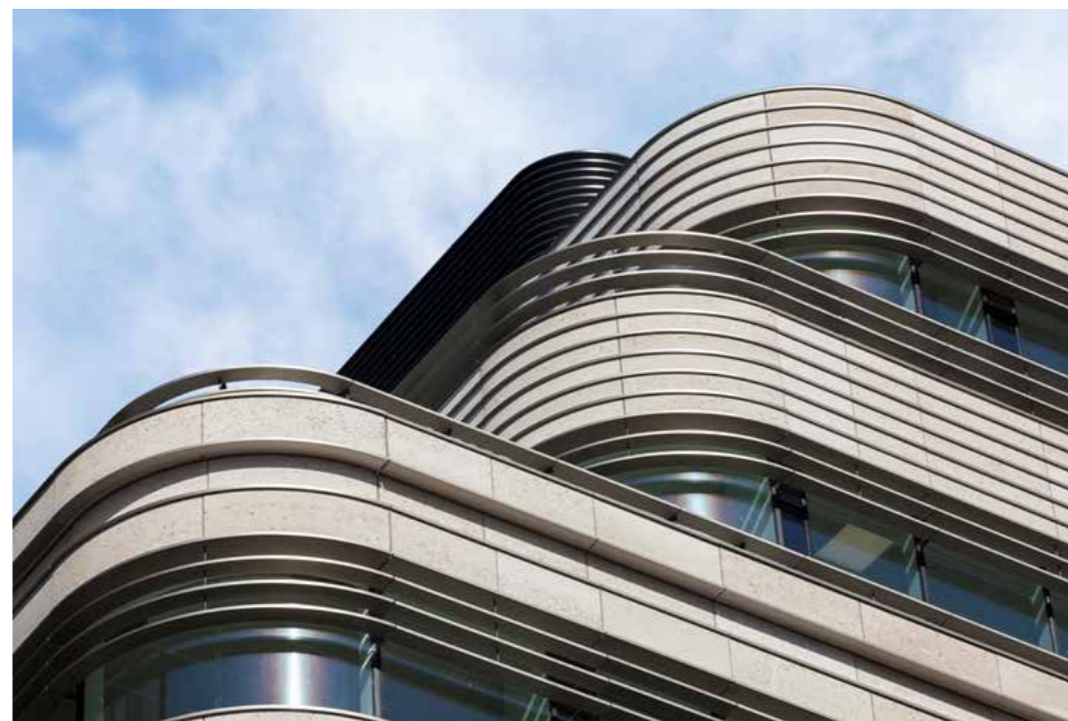
Horizontal running cladding, St. James' Market, London
