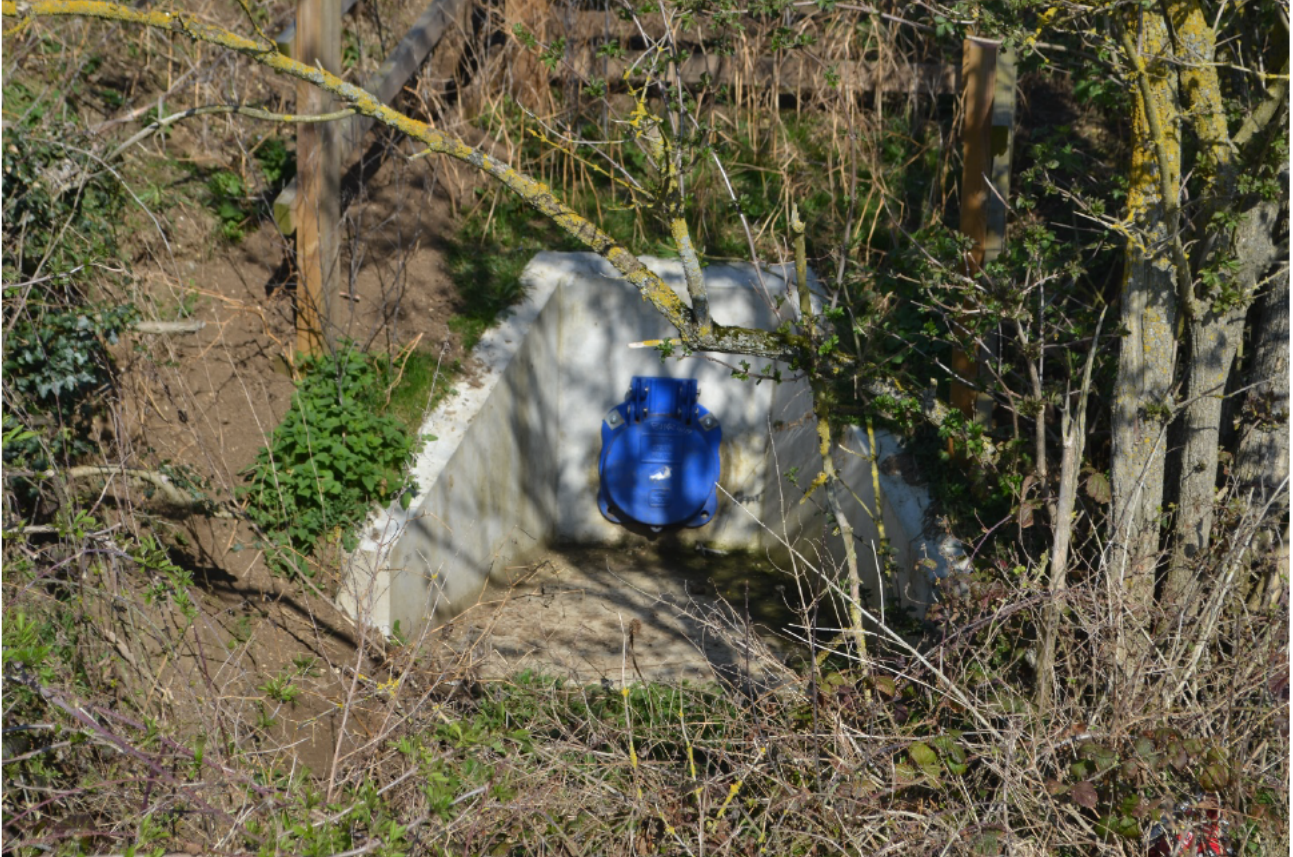
Photograph 6.3: The Kingfisher Pond overflow pipe, March 2021
