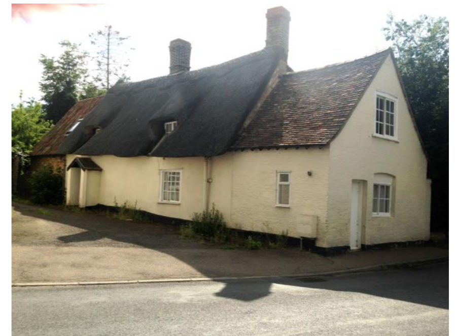
Figure 31: view looking south towards 63 and 65 Pierce Lane from the north side of Pierce Lane.
