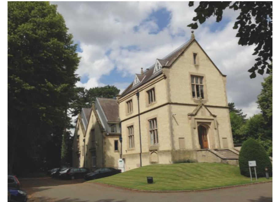
Figure 33: view looking north-east towards the Former Pumping Stations at the Cow Lane (southern) frontage.
