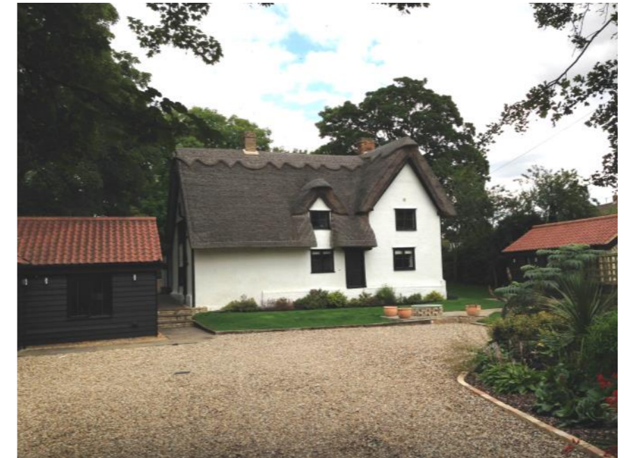
Figure 30: view looking east on a backland site lying to the north of Cow Lane showing 28 Cow Lane.
