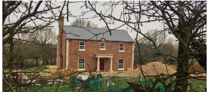
Fig 29 New house nearing completion, Little Heath
