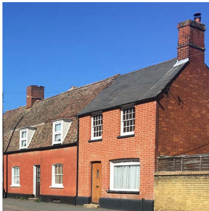
Fig 59 Church Street cottages
